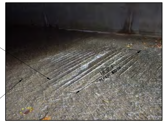
MP 174.71 FLOOR SLAB AT SOUTHWEST QUADRANT
