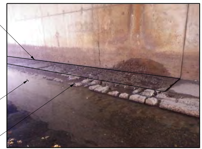
MP 179.76 TOP OF FOOTING ALONG EAST ABUTMENT
